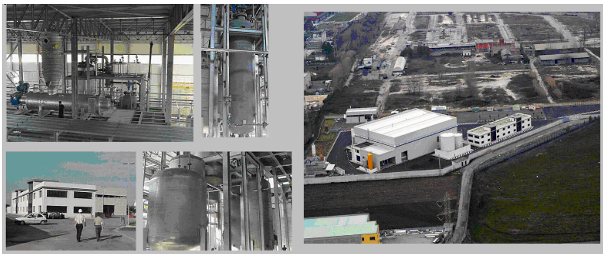
Figure 1.3 Plant in Caserta (Italy) for the production of levulinic acid and ethyl levulinate. Storage tanks (top left); exterior of the building (bottom left); mixing tank (top center), the second reactor (bottom center) aerial view (right).
